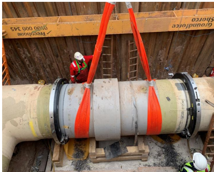
48" IJ Removal in Progress
